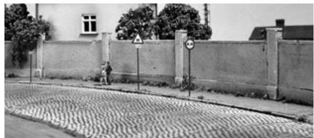
Above: Cobblestone road built with large radius casts from mould 1023 and sidewalk mould 1073 or 1075. Rough cast walls from mould 7024.
