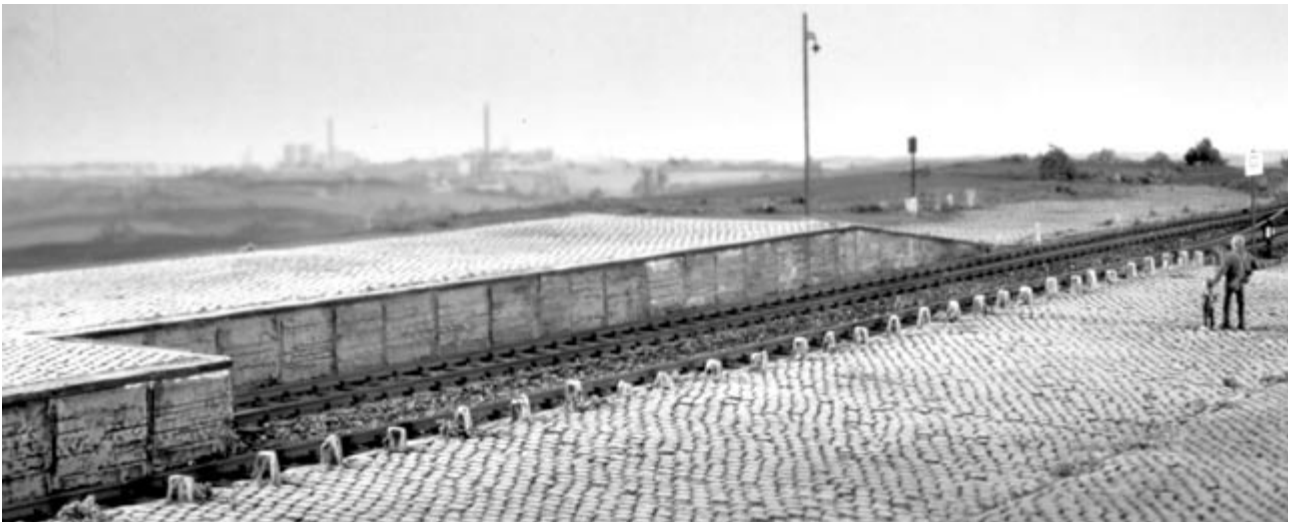
Cobblestone load street (mould 1006) and freight ramp with concrete base wall (1050) and ramp surface of cobblestone (1005).
